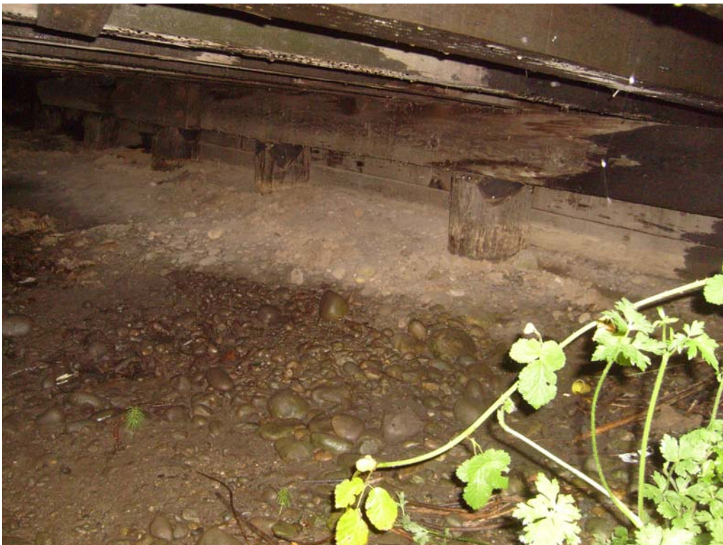
Photo No. 6: Pier 3 looking northwest.
