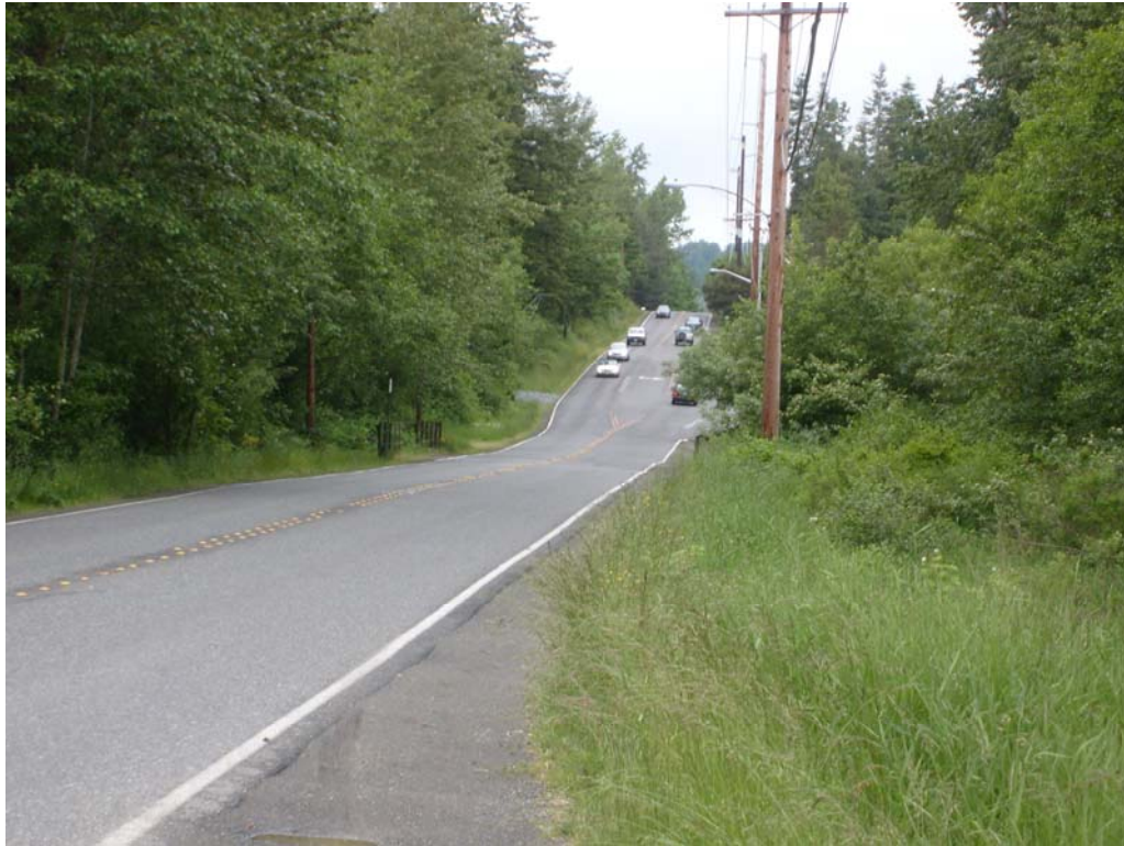
Photo No. 1: Roadway Deck looking north.
