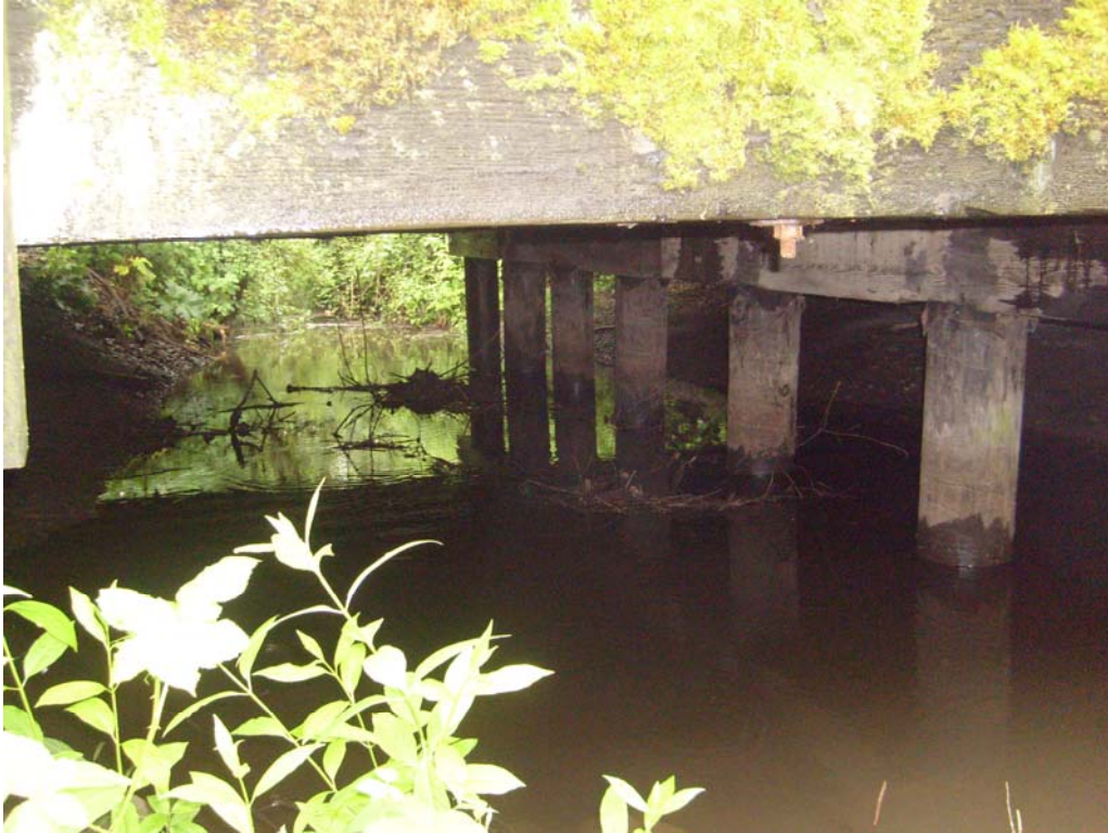
Photo No. 5: Pier 2 looking northwest.
