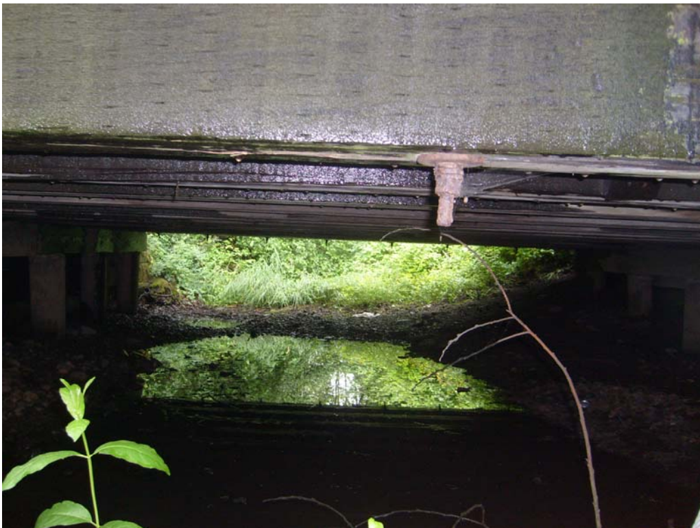
Photo No. 4: Elevation looking west.
