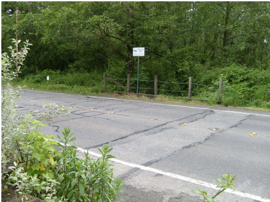
Photo No. 2: Roadway Deck looking southwest.
