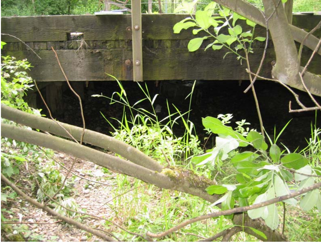
Photo No. 3: Elevation looking west.
