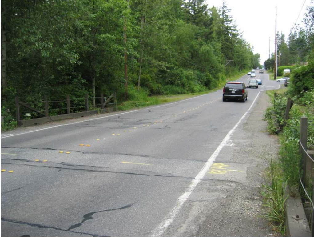
Photo No. 1: Roadway Deck looking north.
