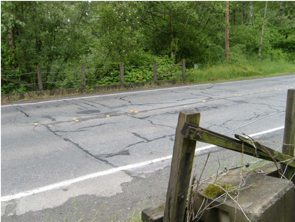
Photo No. 2: Roadway Deck looking northwest.
