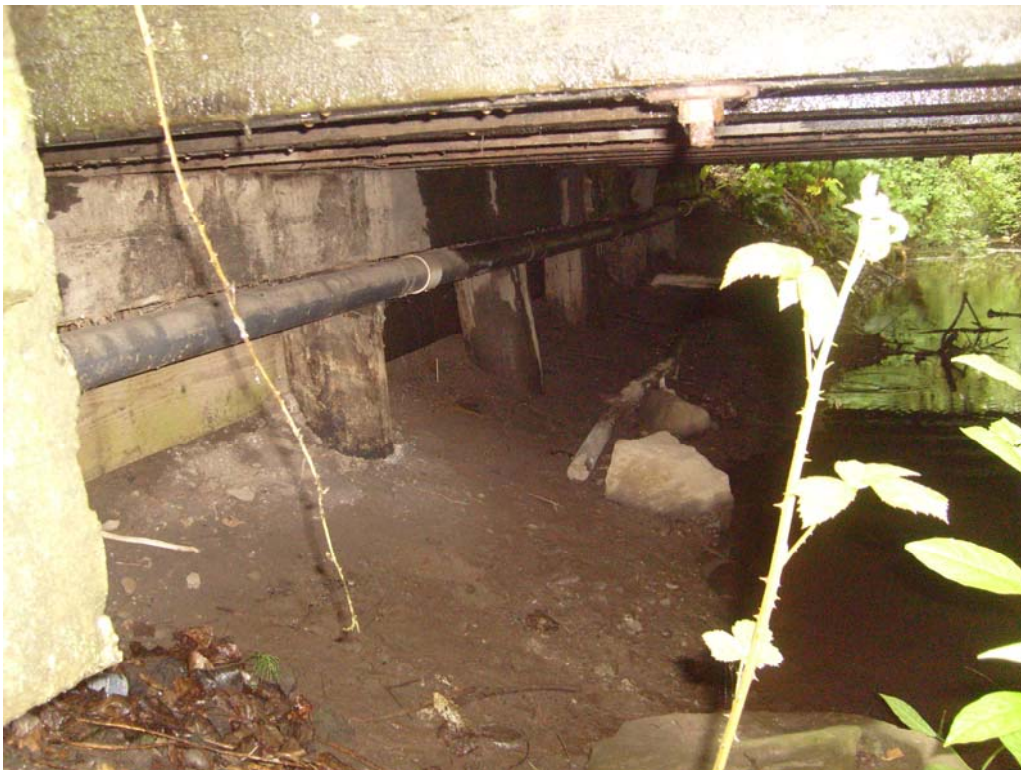
Photo No. 4: Pier 1 looking southwest.
